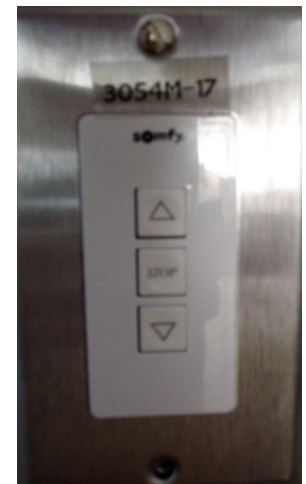
There's also a wall-mounted control for the screen
